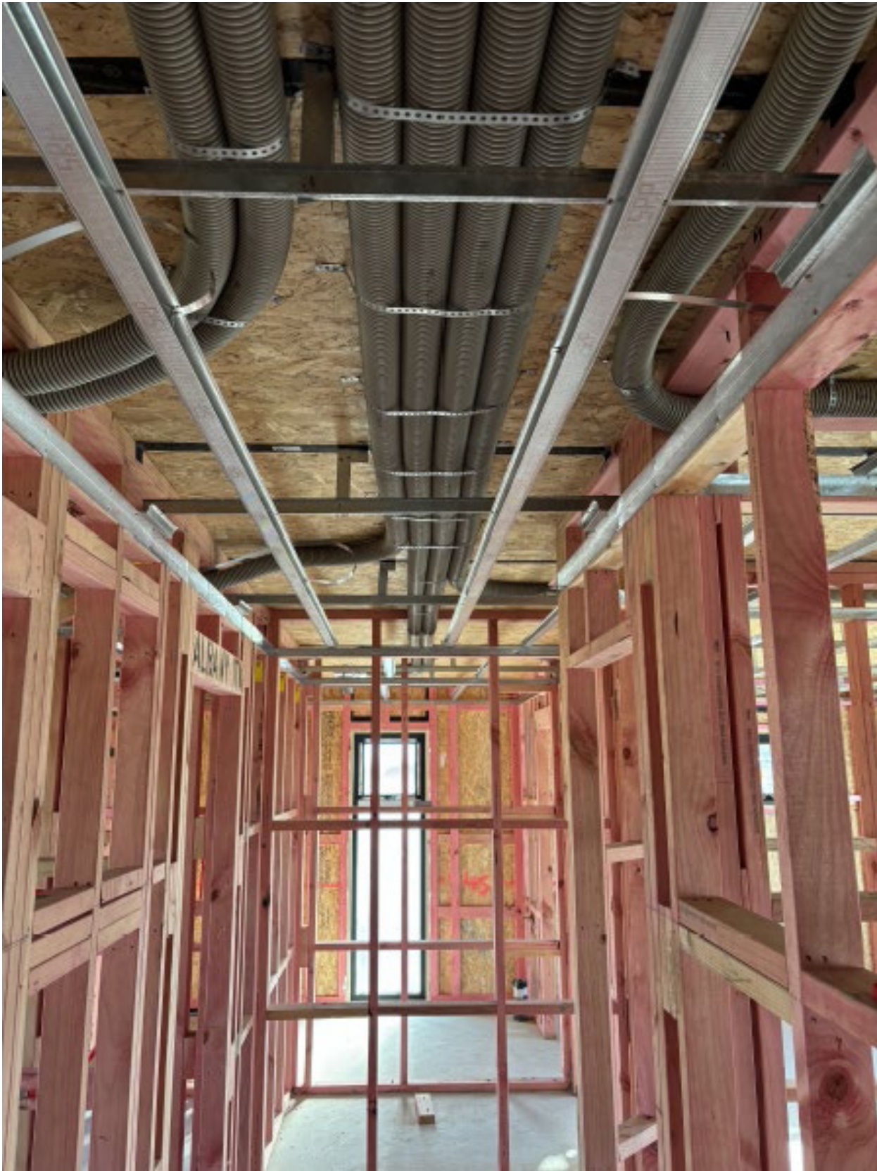
Example of top plate construction for service cavity
